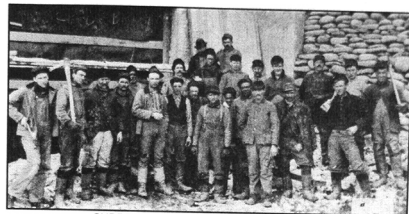
CUDDERBACKVILLE HYDRO-POWER PLANT
